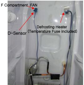
[Location of Connection sockets of Freezing Compartment Electronic Units]
