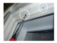
Open the Hombar Door and unwind the fixing bolts of the Ledge Cover at the top.
