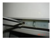
Remove the fixing bolt of the Ledge.
