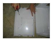
Loosen screws at bottom of a changing room cover.
