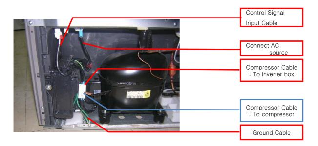
3-2) Check method for compressor terminal of compressor malfunction.
