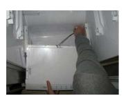
Lift up a changing room lightly and pull it forward a little bit and separates a housing and then separate a changing room.
