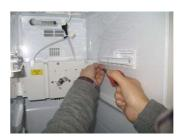
Loosen 4 fixing screws for a Geared-Motor box.
