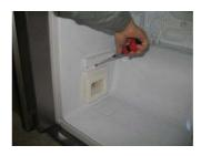
Loosen a screw of a damper cover assembled at left side of a refrigerator.
