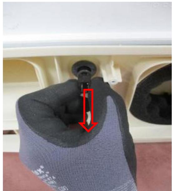
1. Remove NTC sensor socket.
