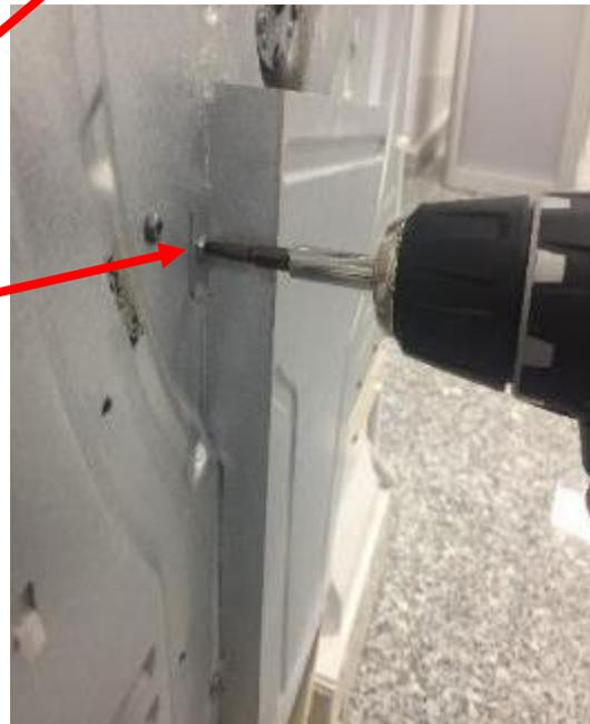
1. Remove 4 screws of air guide bracket located under the heater
