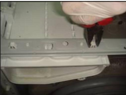
1. Remove the tub seal clamp by using the pliers, which is attached to the detergent drawer housing.
